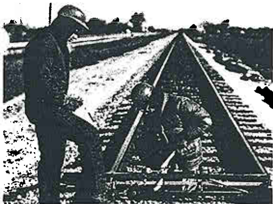
Inspection of ties in Lorenzo, Illinois test track.
